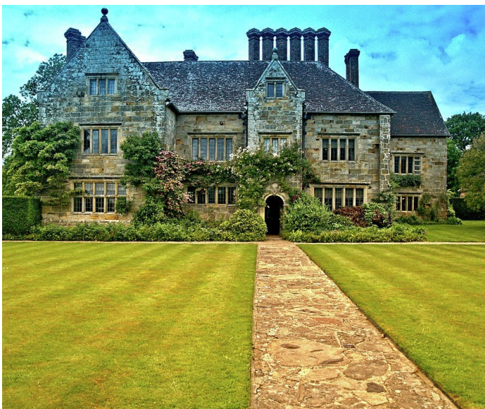
Below — Bateman's in the sunshine!
